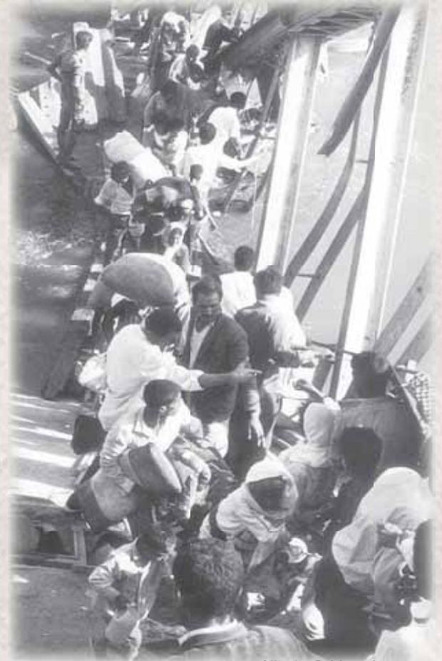
Allenby Bridge, June 1967
