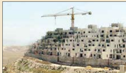
Ongoing construction at Ma'ale Adumim
