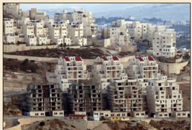
Ongoing construction at Har Homa
