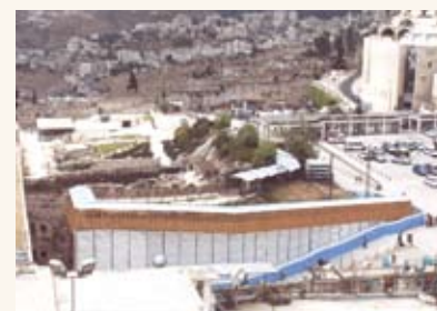
Recent excavation near Mughrabi Gate
