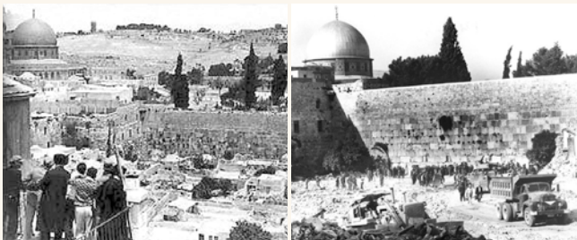
The Moroccan Quarter in front of Al-Buraq Wall prior (l) and after (r) its demolition.
