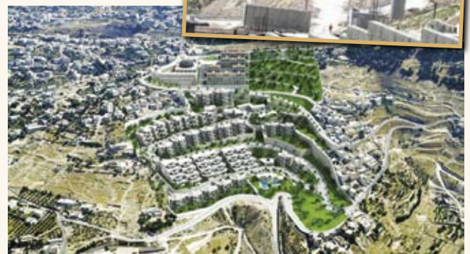
Nof Zion: Completed settlement as advertised on the project's website (Jabal Mukabber in the background); small photo: ongoing construction at the site.
