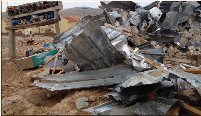
Home demolition in Um Al-Kher, West Bank
