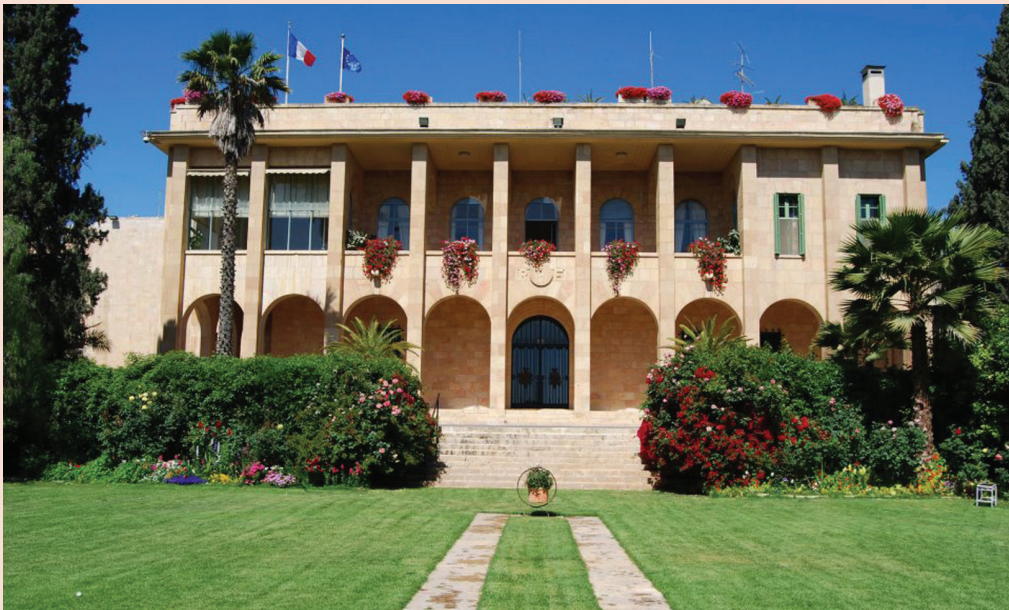
French consulate general - consular and diplomatic section - in Jerusalem, located west of the Green Line
