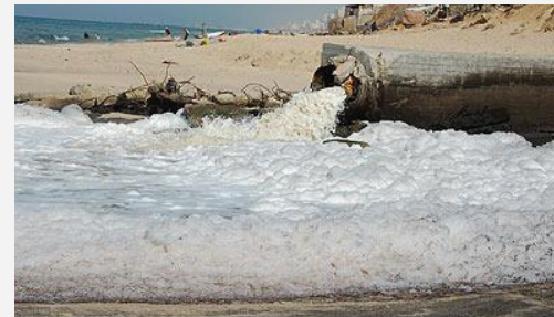
Raw sewage discharged into the sea
