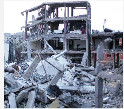
Destroyed residential area
