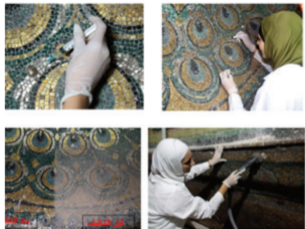
Hashemite restoration of the mosaics in the Dome of the Rock in 2008 until June 2016.
