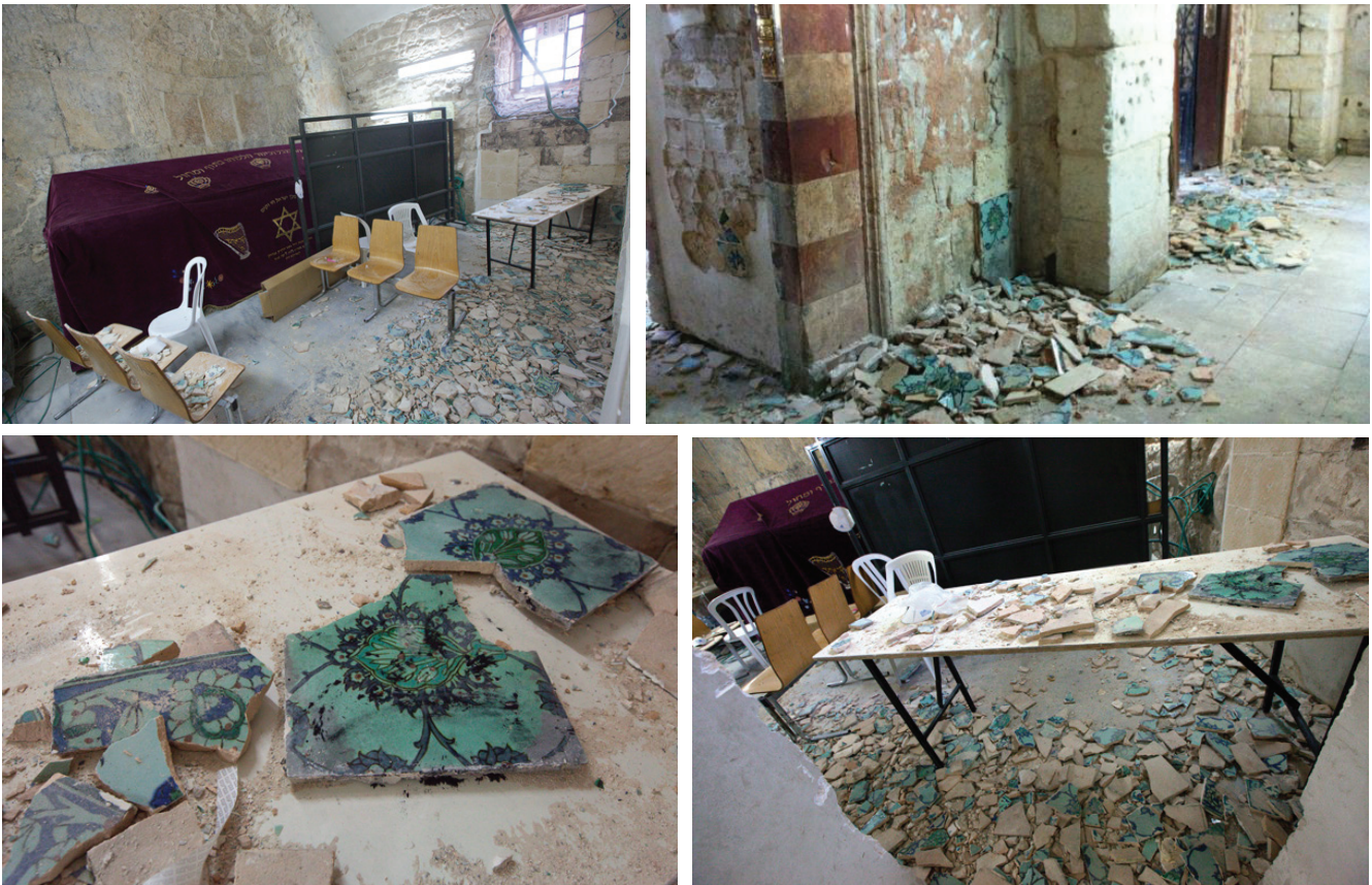
Documented damage at Nabi Dawoud Mosque.
