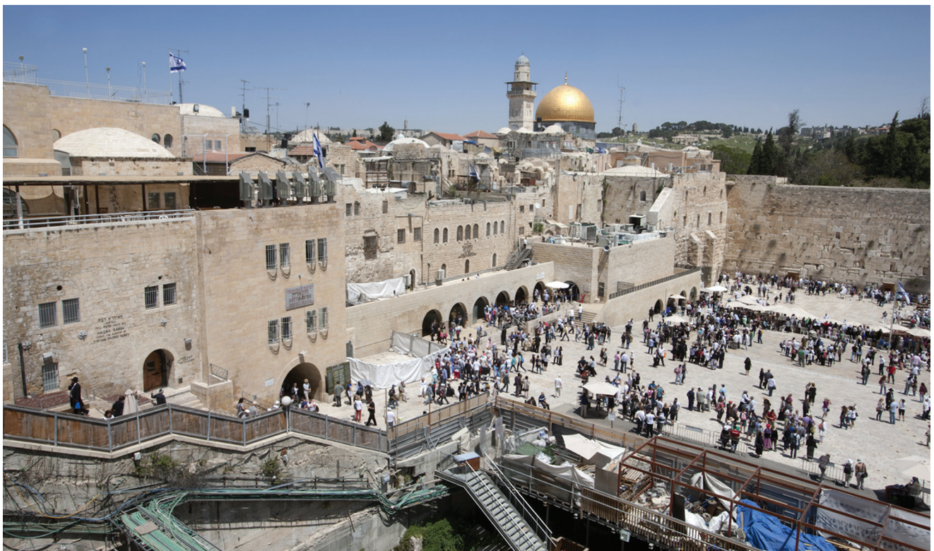
Demolitions for the construction of Beit Strauss on Muslim Waqf real-estate, 2013-2016
