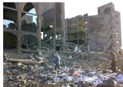
Houses in Gaza damaged during Operation Cast Lead
