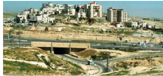
Eastern Ring Road – Underpass at Az-Za'im
