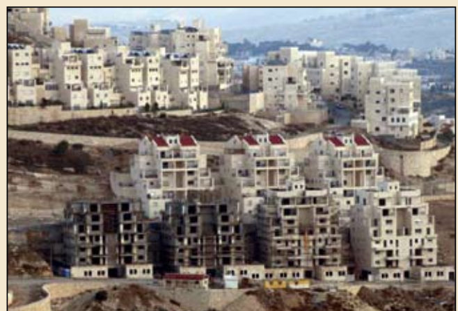
Ongoing construction at Har Homa
