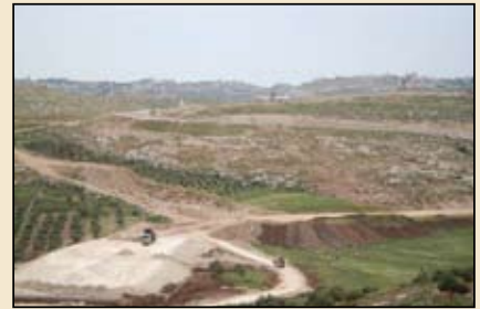
Construction of the Ring Road
