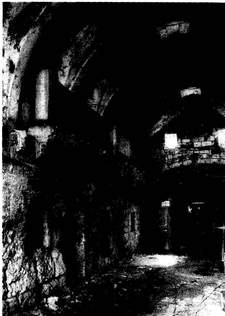
Khan al - Sultan (al - Wakala) entance in Bab al - Silsila Rd. (before restoration)
