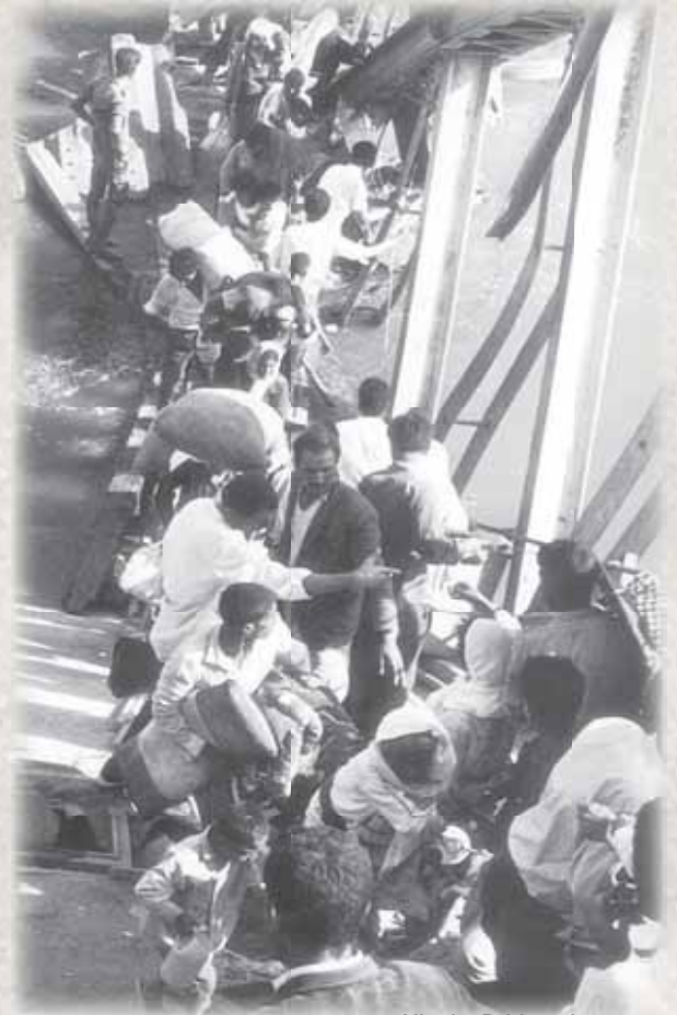
Allenby Bridge, June 1967
